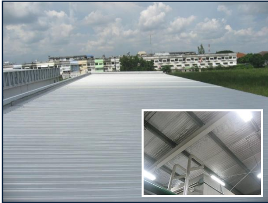
Above: 609m 2 warehouse's roof before painting Caption: existing aluminum foam insulation.
