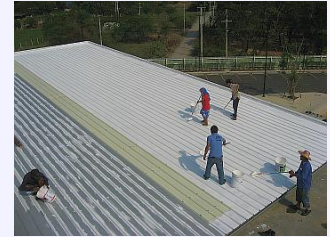
Above: in Japan, a warehouse's air-conditioning system was set to maintain a 25°C temperature indoors. As soon as the rooftop was coated with Planet Supra, the air-conditioning's workload dropped by 20.6kW, a direct 63% saving on electricity cost.
